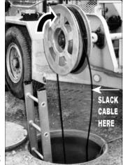
P/N 15472 is a capstan equipped with an integral torque limiter between the driving spindle and the inner hub. The torque limiter limits the pulling tension to a calibrated maximum that has been set at the factory to 600 pounds-force (2669 N).
